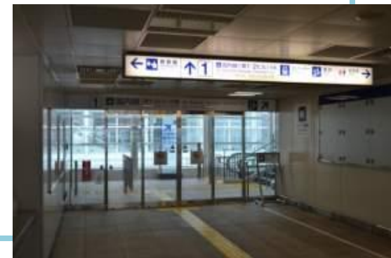
Doors installed by the monorail ticket gates
